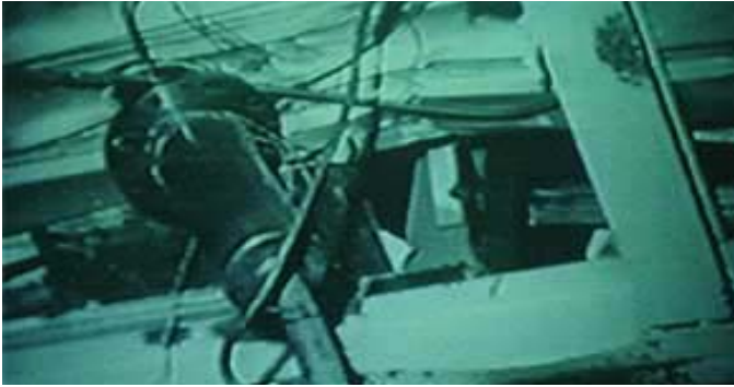
Control rod lodged in ceiling of SL-1 reactor building.
